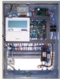
The DX kit enables connection of a third-party party air handling unit (with DX coil) to Toshiba LC outdoor units.
